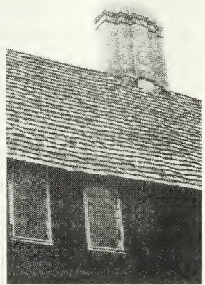
The finished chimney
